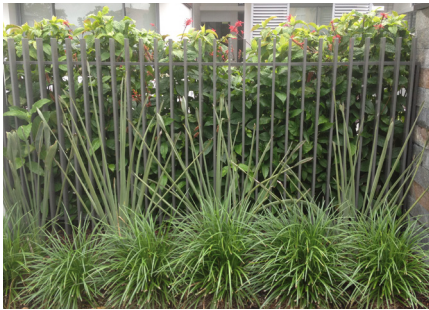
Flat Bar Fence and Gate
